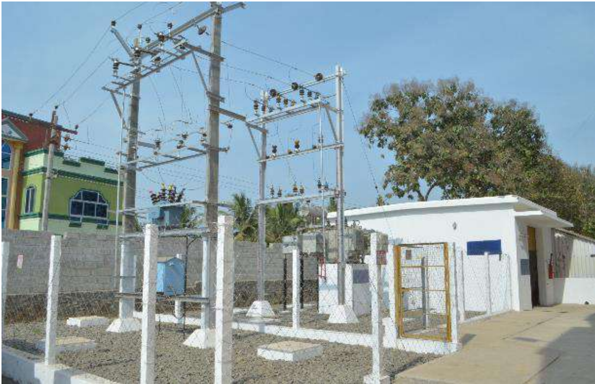
11 kV/415 V HT Substation
