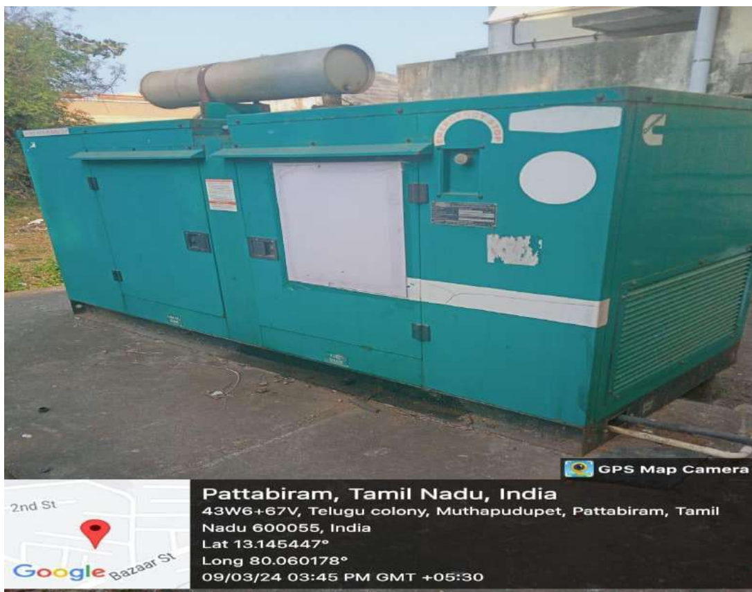
40 kVA Powerica Diesel Generator (1No) installed in our College Campus for Backup Electric Supply
