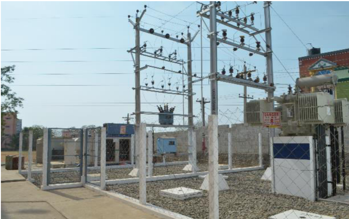
11 kV / 415 V HT Substation
