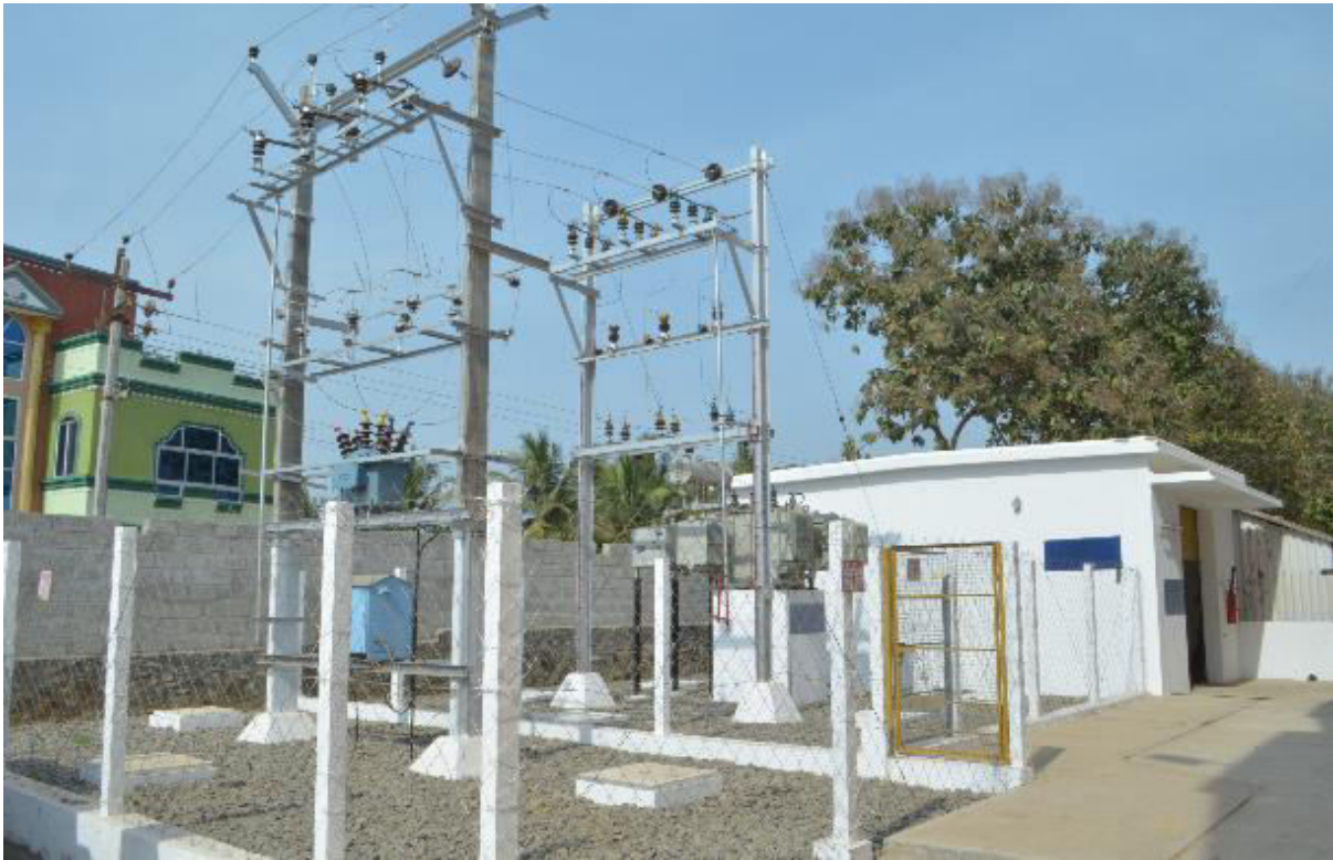
11 kV / 415 V HT Substation
