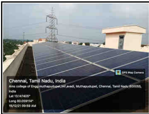
Figure 9.3.3. 20 KW Rooftop Solar Panel.
