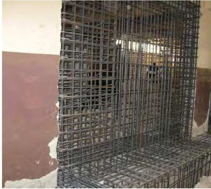
Fig. 3. Infill wall application in an RC building
