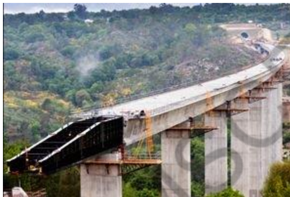
Fig. 2: Incremental Launching Box Girder Construction Method
