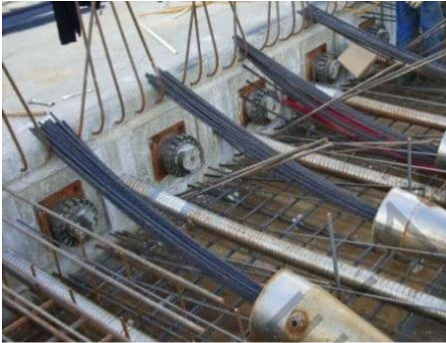
Fig 4: Arrangement of Tendons Before Concrete Filling In Post Tensioning Method of Bridge Construction
