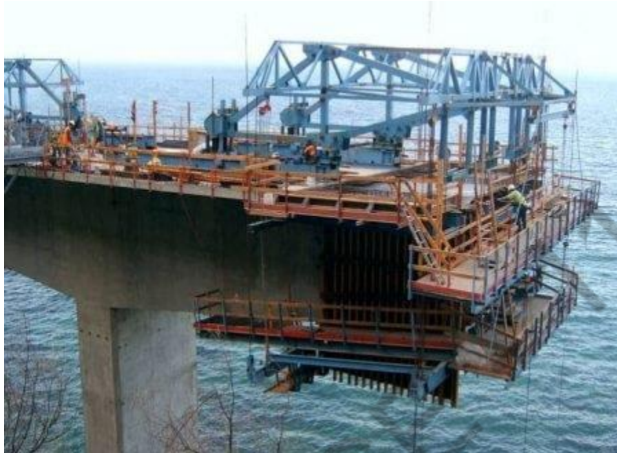
Fig 3: Cast-in-situ Balanced Cantilever Method of Construction
