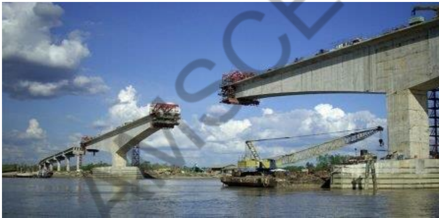
Fig.1: Balanced Cantilever Bridge Construction
