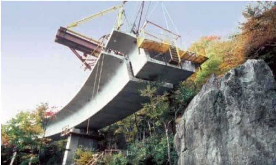
Fig.2: Precast method of bridge construction
