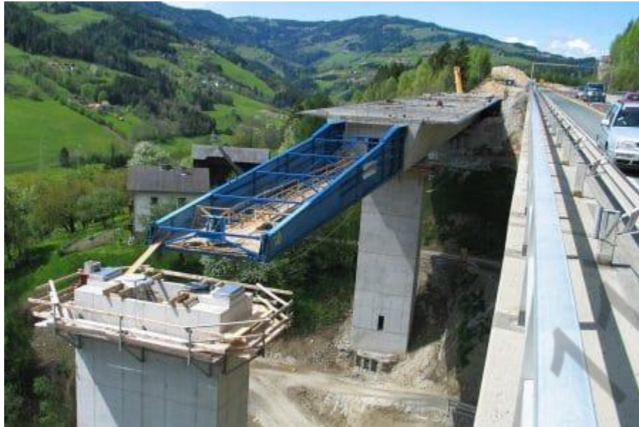
Fig.3: Incremental Launching Method of Bridge Construction
