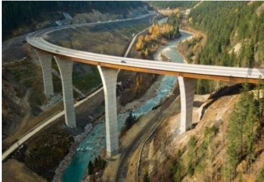
Fig 2: Bridge Constructed Using Cast-in-situ Incremental Launch Method
