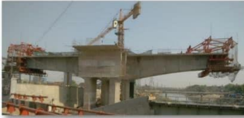
Fig. 1: Cantilever Construction Method for Box Girder Bridge
