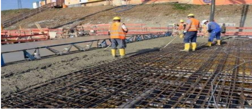
Fig 5: Cast-in-situ Concrete Filling
