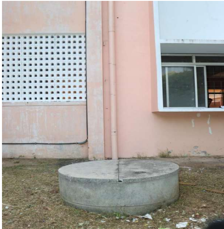
Recharge pit on campus grounds
